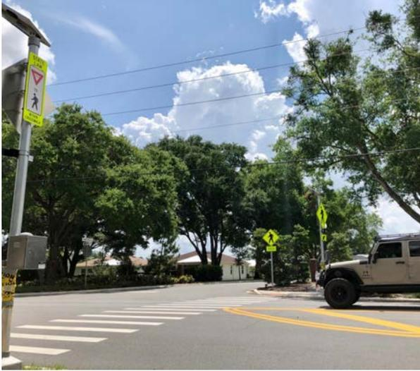
As a pedestrian safety measure, the Town has installed a crosswalk, signage and a rapid-flashing beacon at the mid-block crossing on Oakland Avenue near Sansparilla Road.
